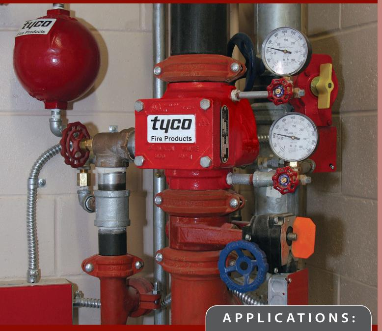
Wet Pipe Sprinkler Systems are designed for use in applications where the temperature is maintained above freezing. In such systems, the entire piping network is fully pressurized so that water is discharged from a sprinkler head immediately after actuation.
